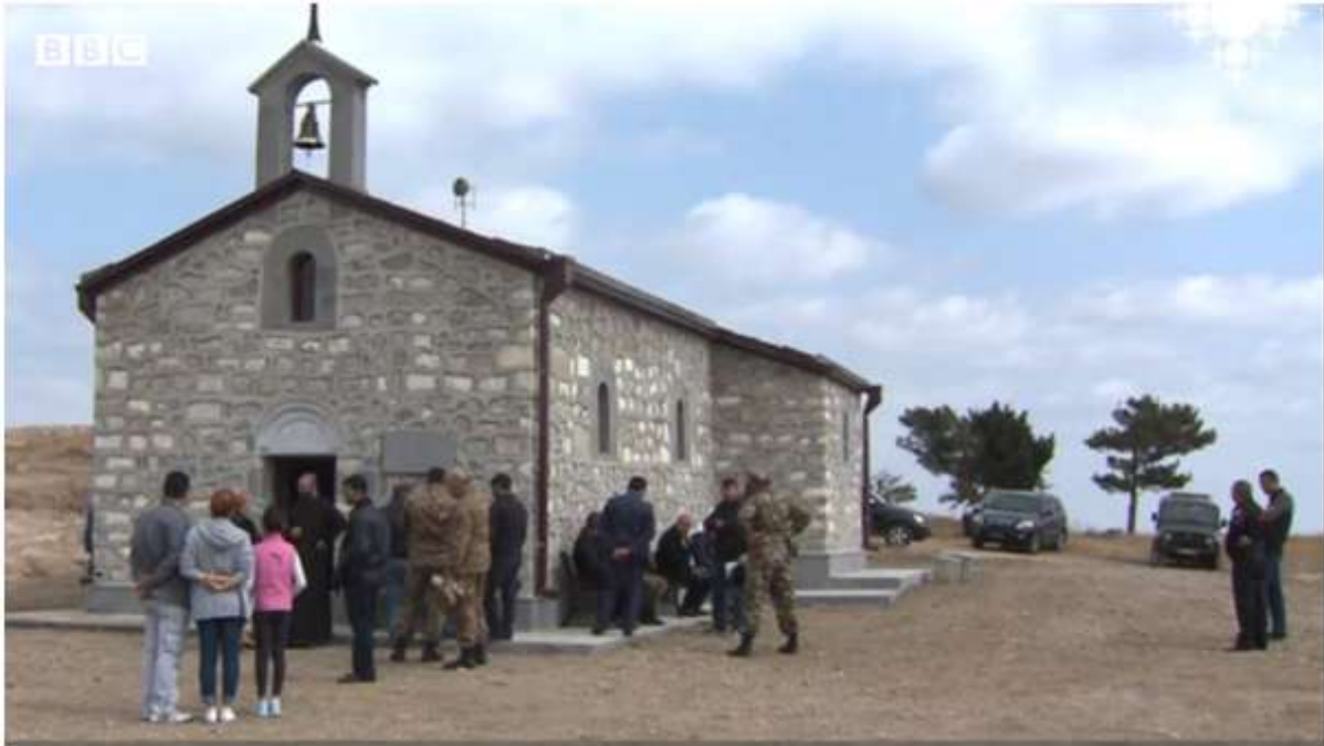
Figure № 7 - Mekhakavan church after it was occupied by Azerbaijani forces on 9 October 2020.
